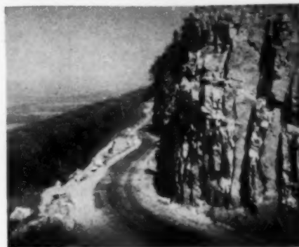
Door to Dade. View looking west toward Sand Mountain. This highway, recently constructed and blasted from solid sandstone beds, connect Dade County with the rest of Georgia.
